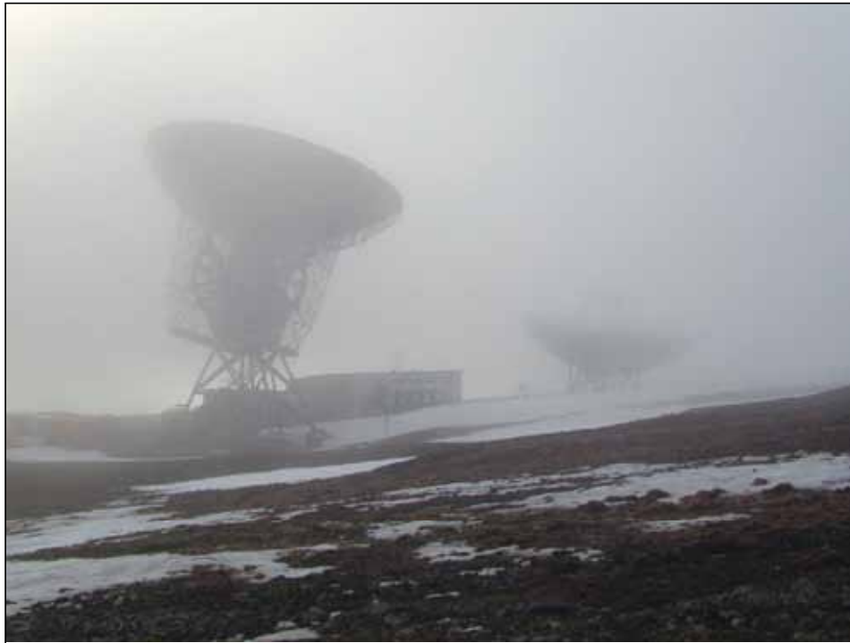
Figure 15. ESR antennas, in the early hours of July 9, 2006. The 32 antenna (left) is pointed towards East, azimuth 90^\circ , at 75^\circ elevation. The magnetic-field-aligned ESR 42 m antenna (right) was not used in the beam park measurement.
